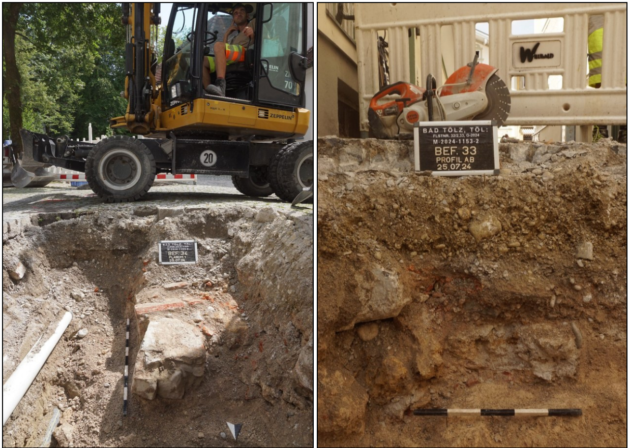
Abb. 27 Links: Fundament Bef. 34. Rechts: Fundament(?) Bef. 33.
